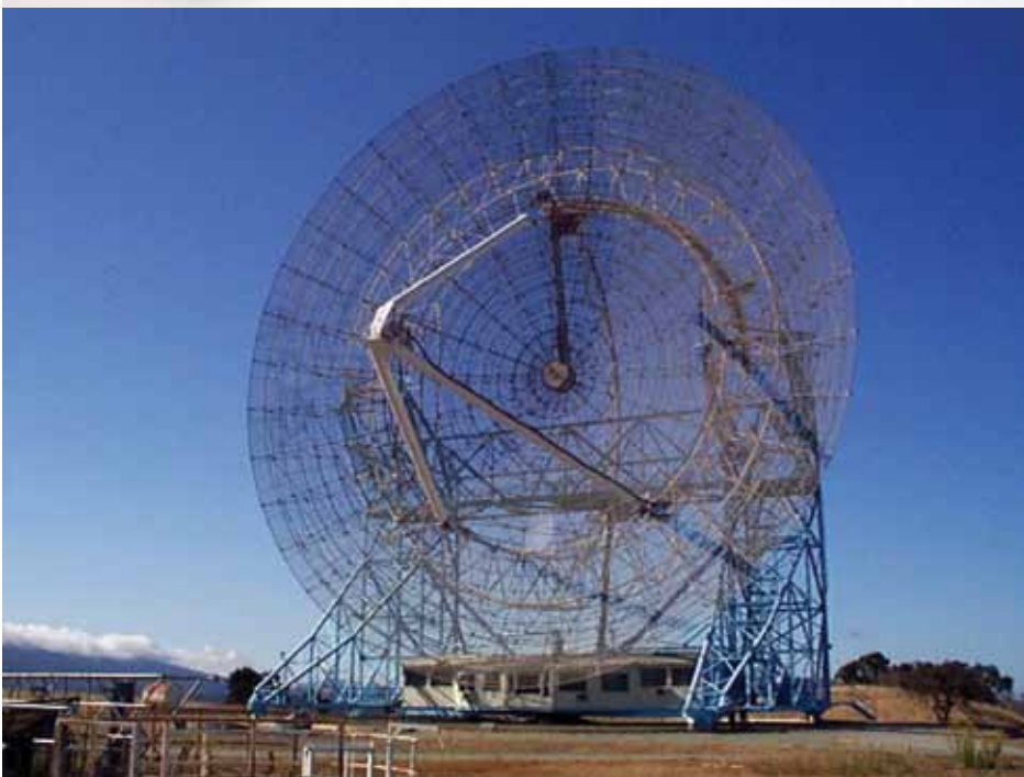
The 250-gram PicoSats (top) and the 150-foot-diameter ground station antenna needed to close the communications link to space (bottom).
