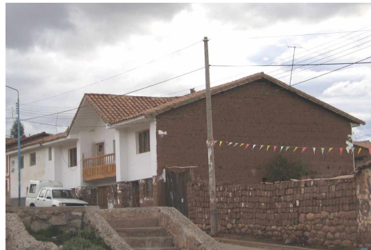
Figure 2. Adobe middle class house in the Peruvian Andes with architectonic and constructive influences from reinforced masonry.
