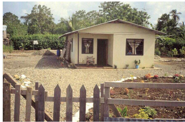
Figure 15. Undamaged bahareque house after the M_L 7.5, 1991, Costa Rica earthquake.
