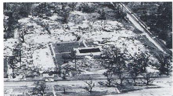
Chauncy T. Hinman The Richelieu Apartments after Hurricane Camille
