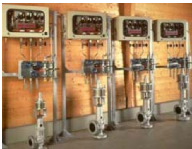
Fig. 9.6.2 Typical supplementary loaded safety valves
