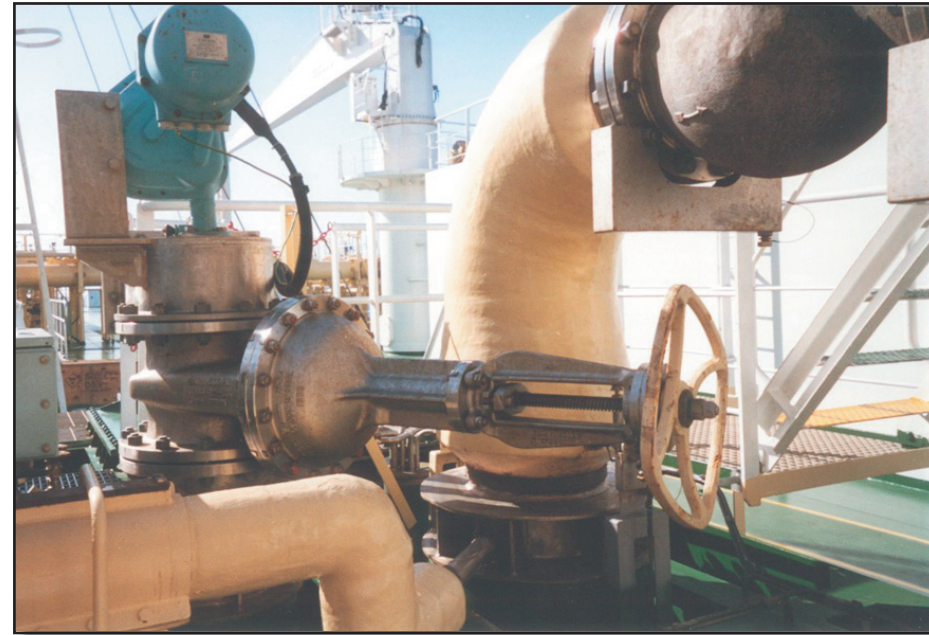
Whessoe Gauge Gate Valve
