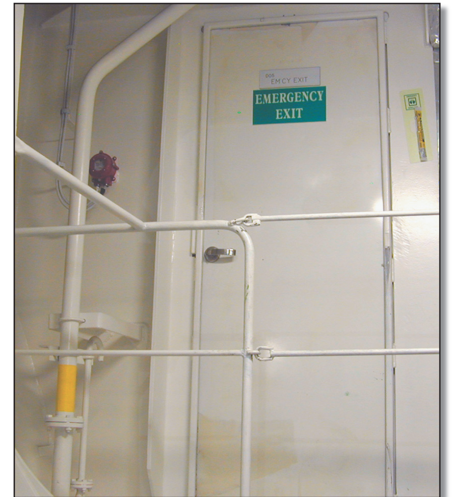
Emergency Escape Door in Engine Room with Emergency Lighting Stick Available
