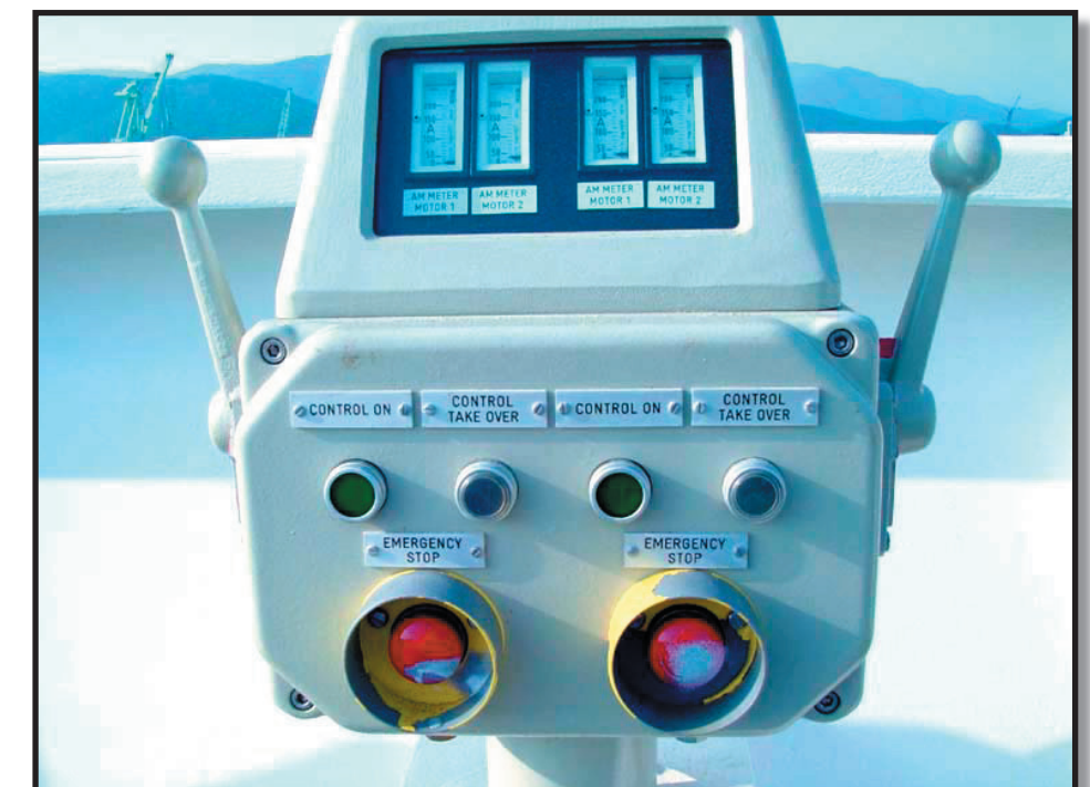
Ship Side Controls
