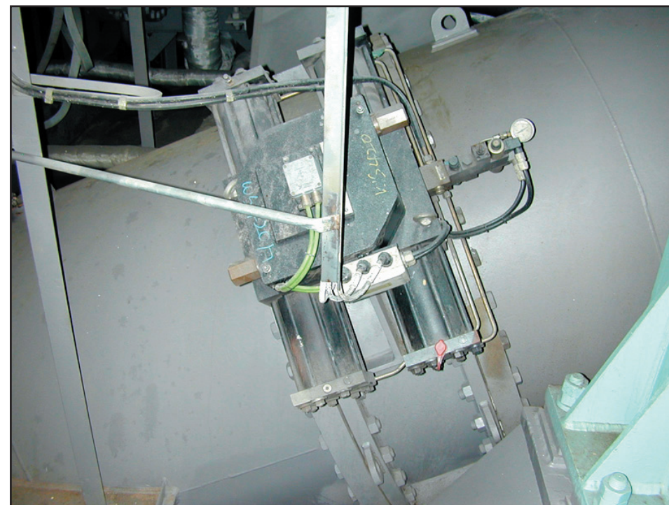
Hydraulically Operated Sea Water Scoop Inlet Valve WS420F
