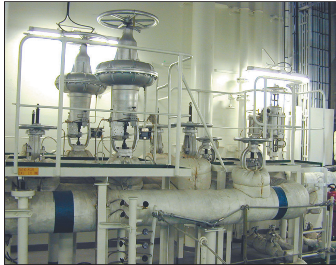
5.88MPa to 0.784MPa PRV DS062F and 5.88MPa to 0.412MPa PRV DS081F
