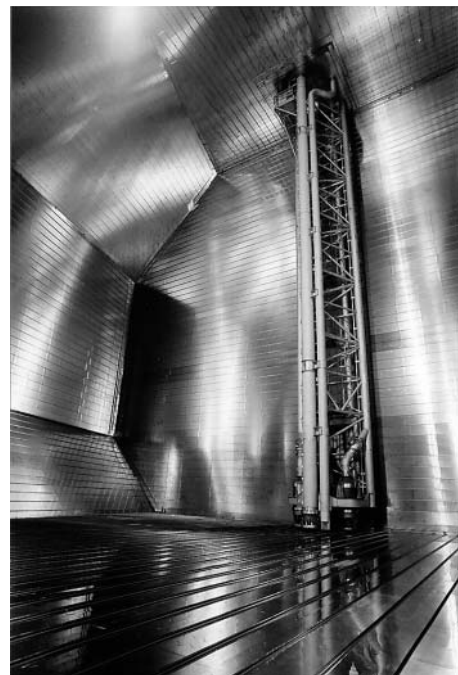
Fig. 12 View of interior of completed cargo tank
